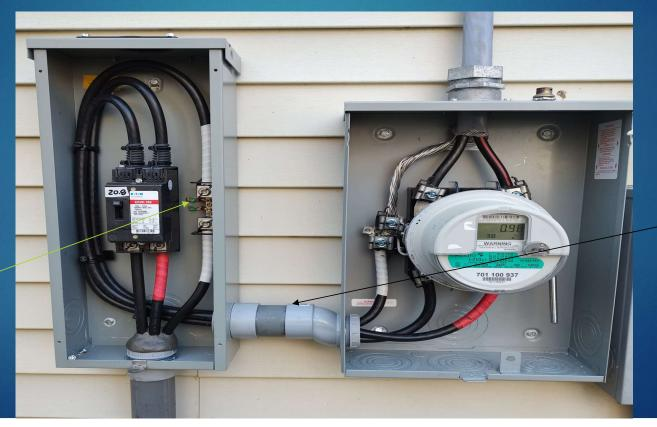
If this conduit is metal, it will need bonding bushings (250.92(A) on each side of fittings and connected to enclosure The utility will provide the AIC rating for the disconnect.
