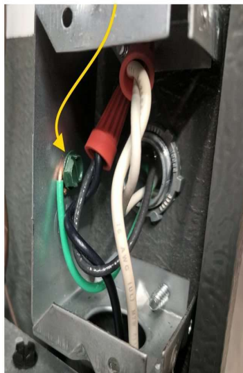
EGC connected to furnace
