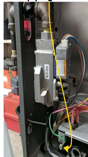
Gas piping bonded
