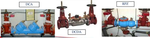
The image shows three different models of water backflow preventers. On the left is a DCA (Double Check Assembly), in the middle is a DCDA (Dual Check with Drain Assembly), and on the right is an RPZ (Reduced Pressure Zone Valve).
