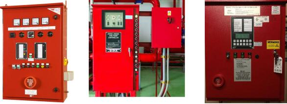
Diesel Pump Controllers
