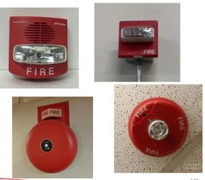
The image shows four different models of red fire notification appliances: a rectangular unit with a speaker and strobe, a smaller rectangular unit, a circular unit with a speaker, and a circular unit with a strobe.
