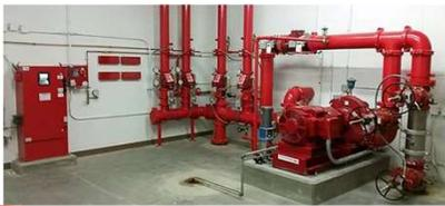
The image shows a large, red stationary fire pump system installed in a room. It includes a main pump unit, various pipes, and a control panel.
