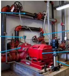
The image shows an electric horizontal split case fire pump with several components labeled with blue arrows:
