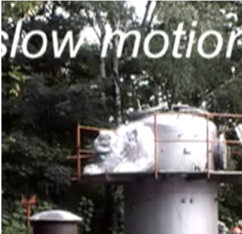
Spring Style – without flame arrestor
