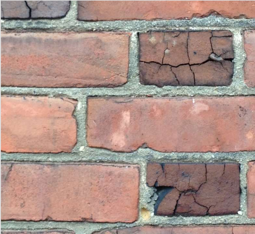
Poor Quality Unit Crack
