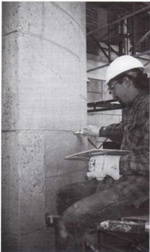
Figure 1. After removing deteriorated mortar, an experienced mason repoints a portion of this early-20th century limestone building. Photo: Robert C. Mack, FAIA.
