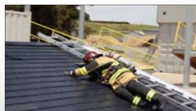
Roof Crews must evaluate for collapse potential and avoid photovoltaic components
