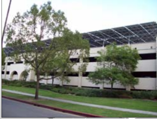
Increased Dead Roof Load
