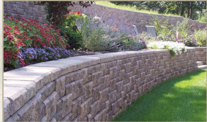
SEGMENTAL RETAINING WALL
